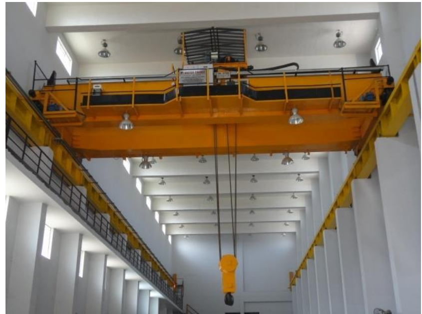
General machinery for magnet development and installed 50 ton EOT Crane .
